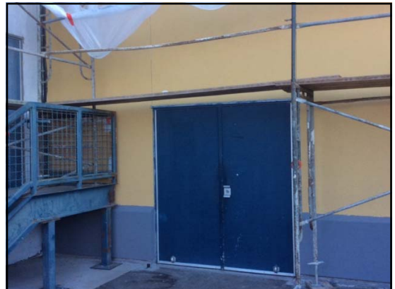
Back North wall with stucco color coat
