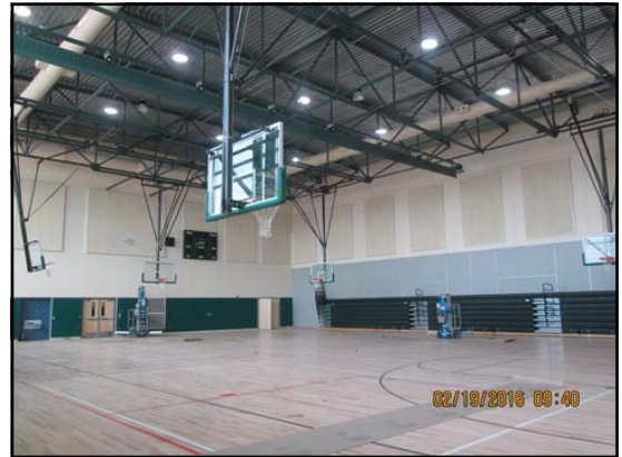
Bldg. B: Gym - Wood Flooring, Bleachers and Wall Pads
