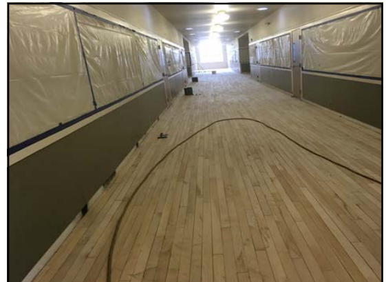
Sanding Hard wood floors in corridors
