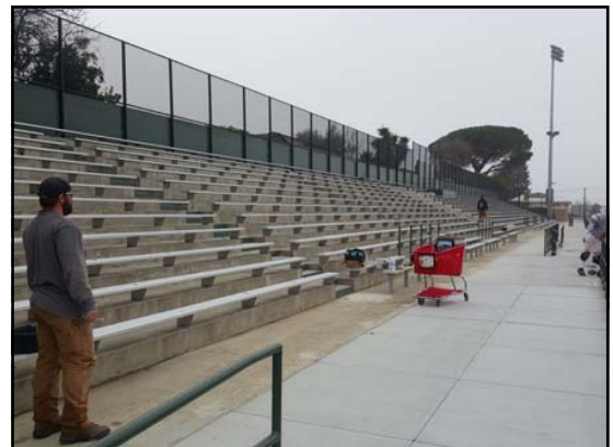
Home Bleachers and Fencing
