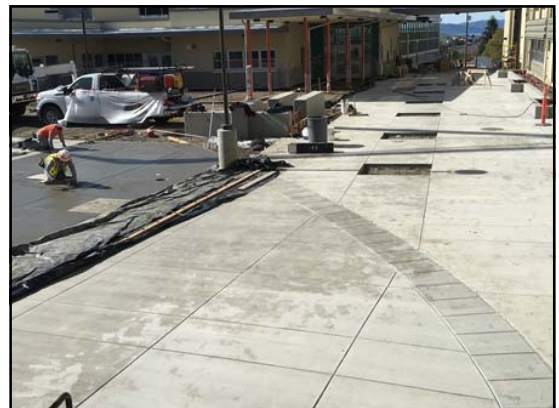
Site: Level 2 - Form, Curb and Flatwork
