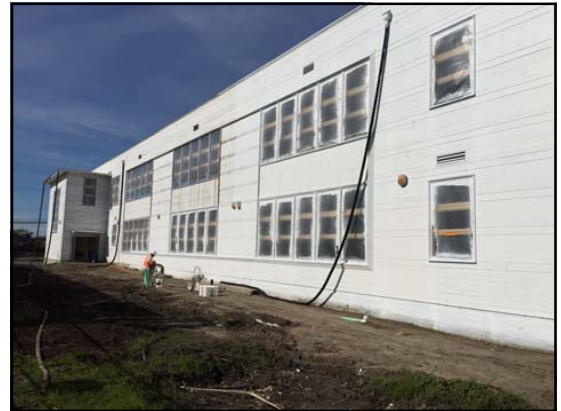
Exterior Painting at Westside
